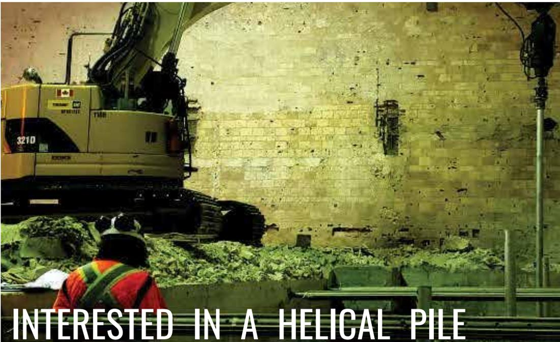
*VersaPile, Inc. installed 64 helical piles to till for Concord Projects inside of the iconic Academy Lanes building in Winnipeg, MB to support its conversion to multi-family condominiums. Air scrubbers were added to the equipment and the supervising engineers were able to monitor the installation torque on their phones using a Wifi connection to VersaPile's Intellitork torque monitoring system.*
